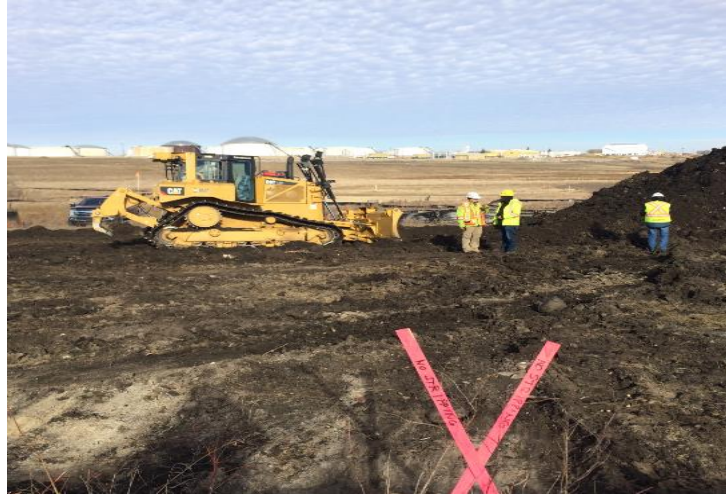
Pipestone Creek ICM's and Archaeologist walk the area excavated
