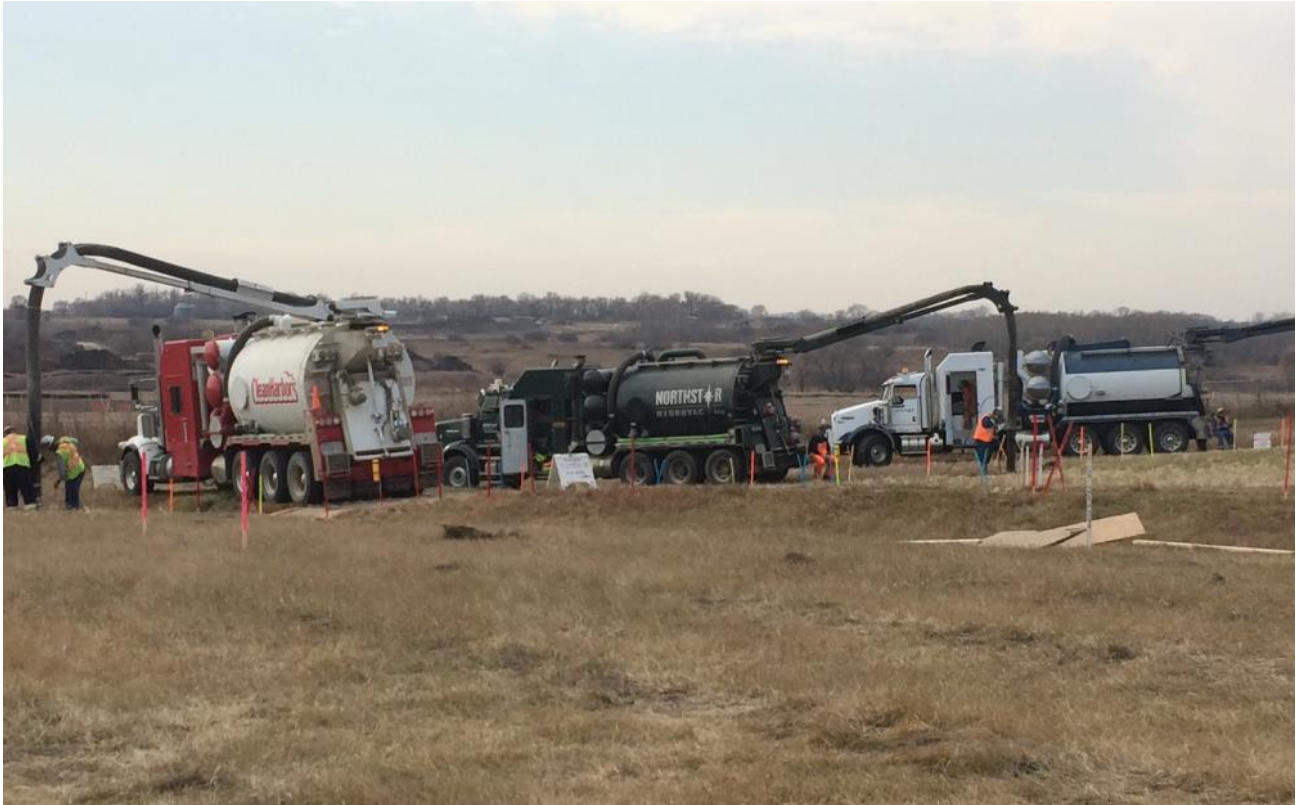
Hydro vacs exposing lines at the Pipestone Creek East side within the Cromer Station
