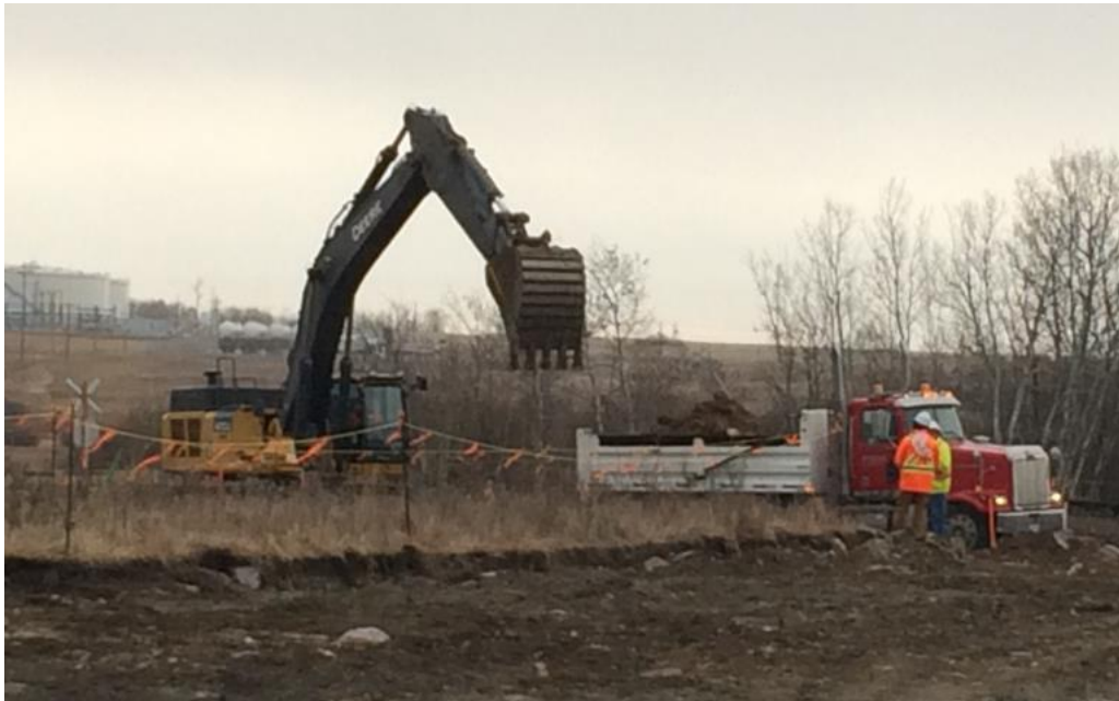
Track hoe digging bore pit west side of Pipestone creek
