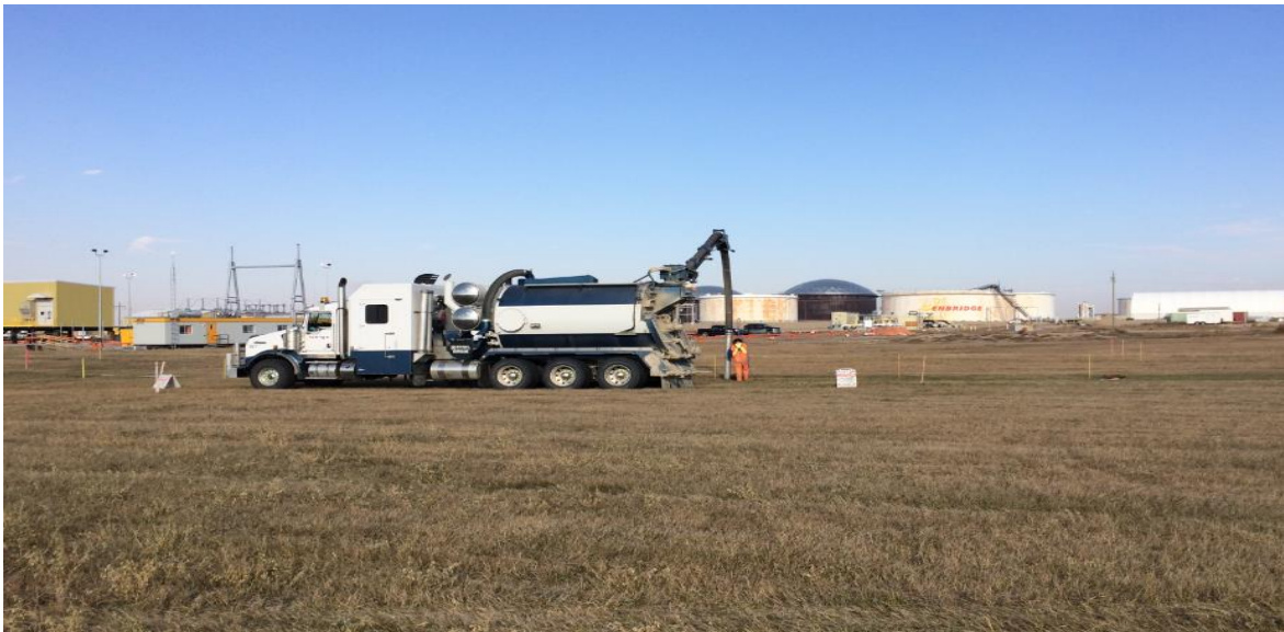
Hydrovac at Outside of Cromer station exposing lines.
