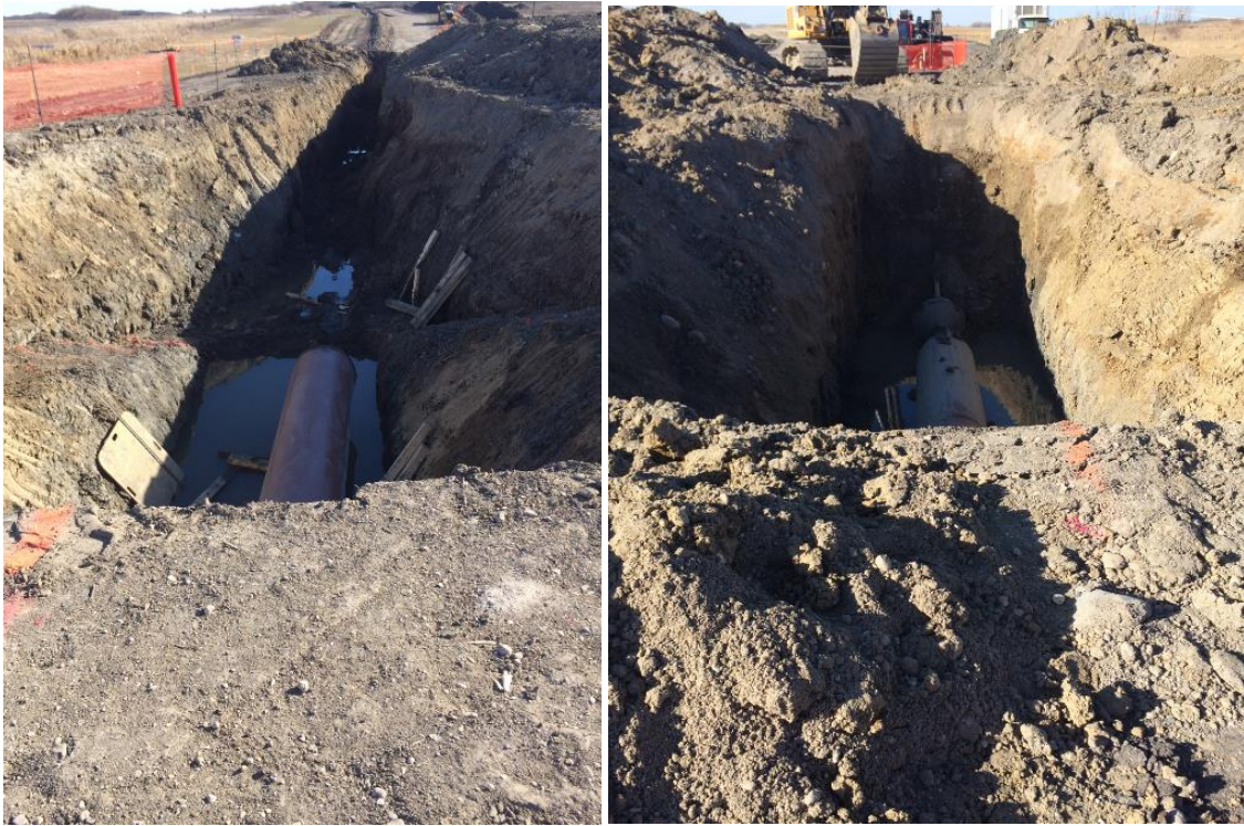
749 + 602 Bore pit excavation
