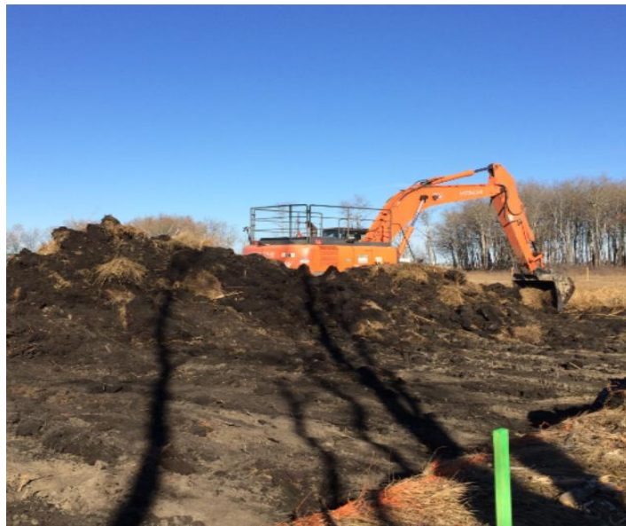
740 + 150 Track hoe pilin clay for ramp across wetland SK 847
